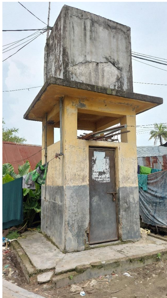
Figure 13: A nonfunctional old water supply tank
