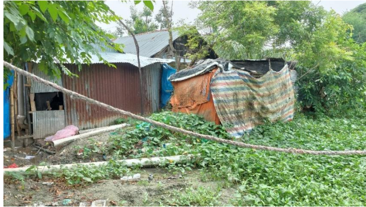
Figure 18: Outlet of human sludge is directly connected to local marshy lands
