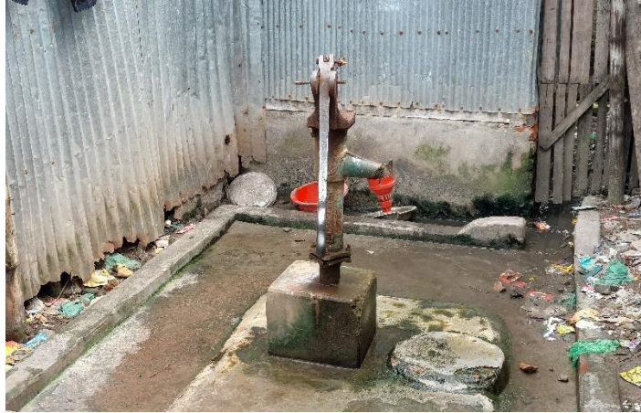
Figure 12: Deep tube well outside the Montu Kaloni
