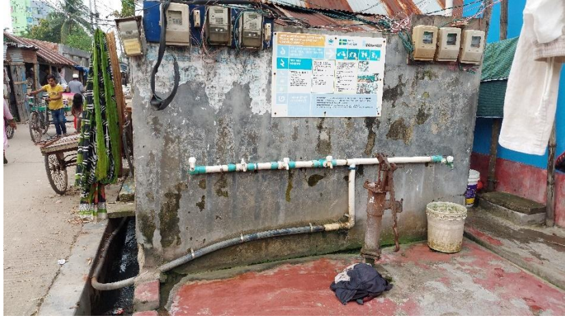
Figure 15: Water supply pipeline from the submersible pump outside Nurani Mahalla
